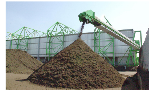
Outdoor composting facility (15.000 t/yr)
